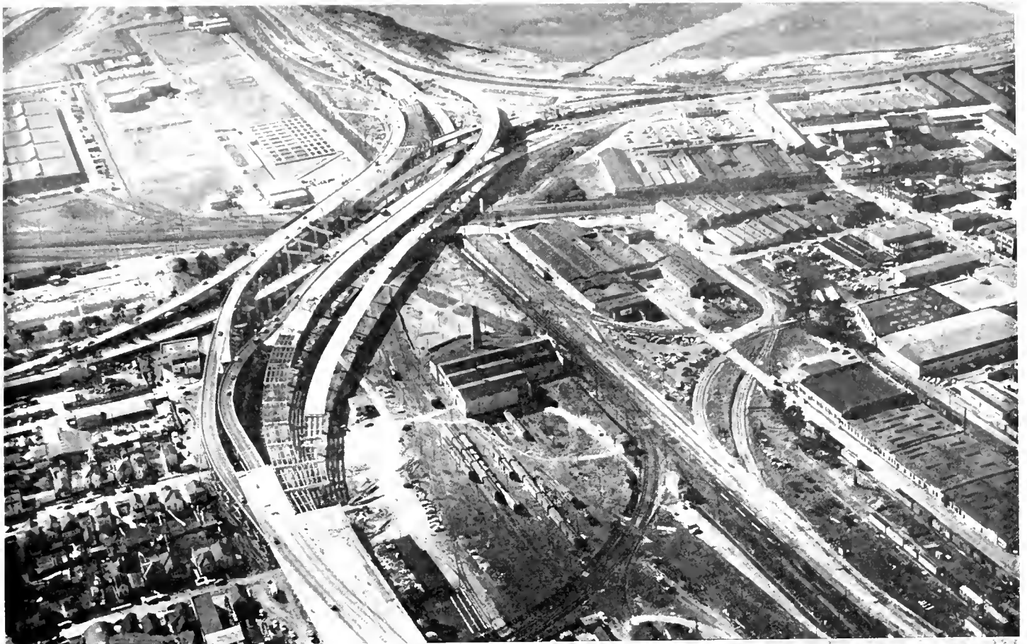
UPPER—Construction operations on additions to the distribution structure looking westerly toward the approach to the San Francisco-Oakland Bay Bridge. The dual two-lane roadways in the lower left of the picture are detours which have been constructed on temporary timber trestles. LOWER—View of construction operations on East Bay Distribution Structure looking east toward MacArthur Boulevard.
